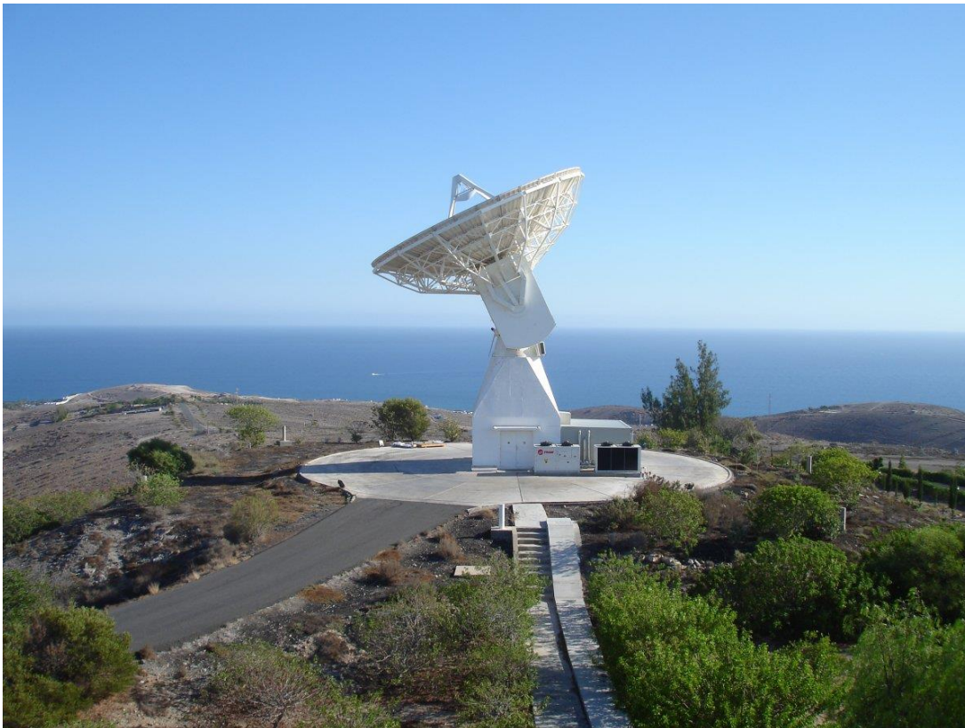
Above: Maspalomas station hosts a 15-metre antenna with reception in S- and X-Band (ESA).
