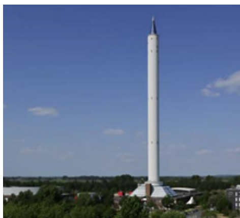
Credit: ZARM; "With a height of 146 meters the Bremen Drop Tower is the only microgravity lab of this kind in Europe"
